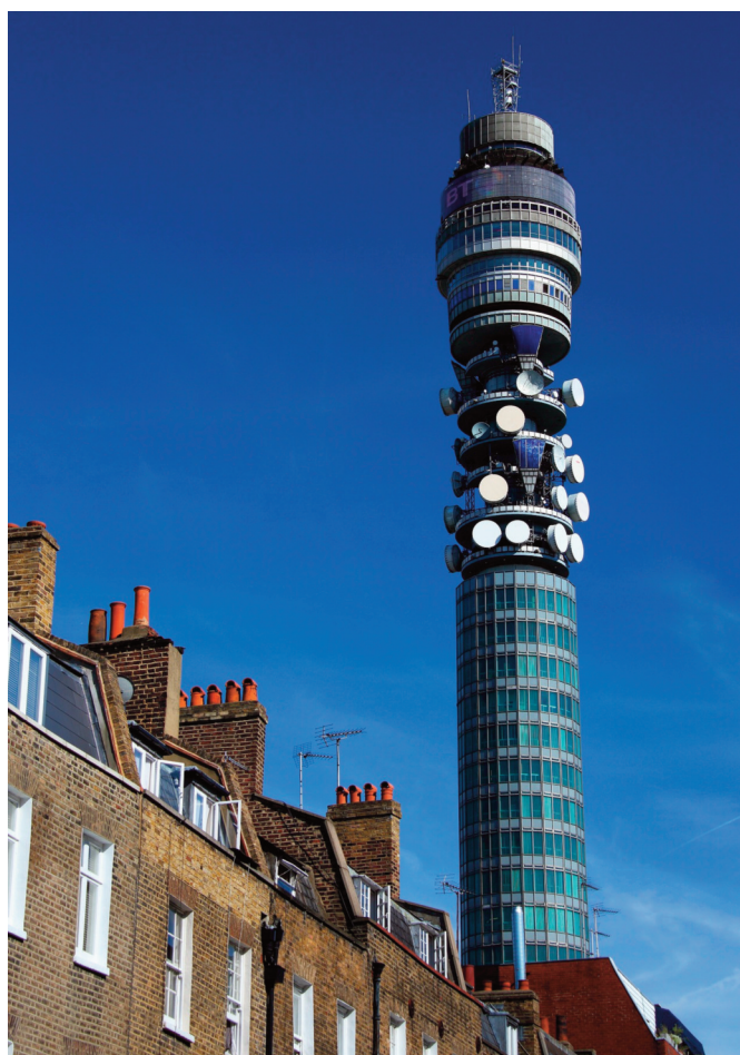
Telecommunications tower in London
